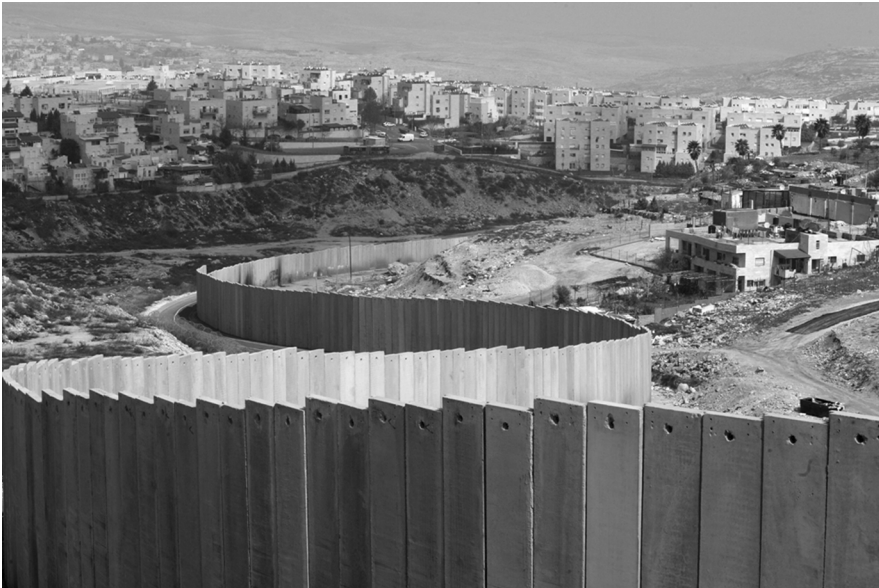
Israel's separation barrier snakes through the East Jerusalem neighborhood of Ras Khamis, where Israeli authorities have handed home-demolition orders to fifty-five families, 4 March 2009. (Ahmad Gharabli/AFP/Getty Images)
